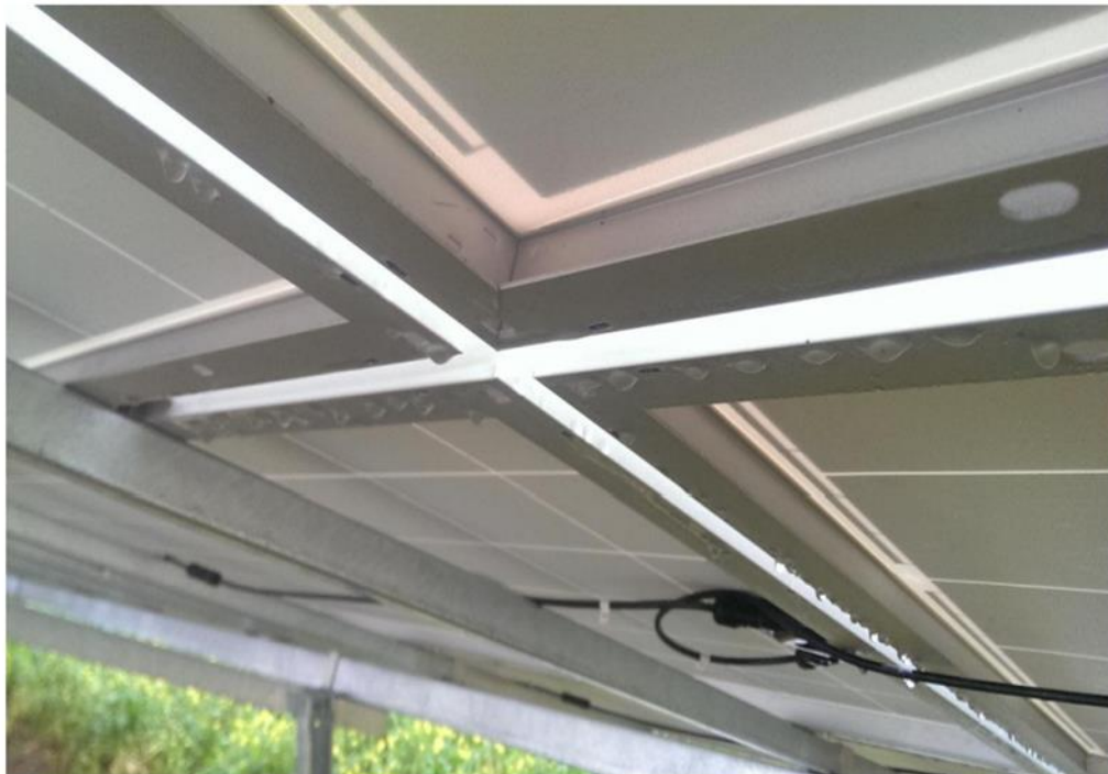
Figure 7. Typical Underside of a solar panel
